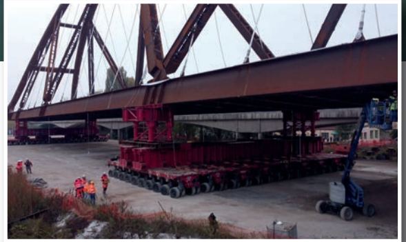
Some 225 lines of SPMT were used to position the bridge.
