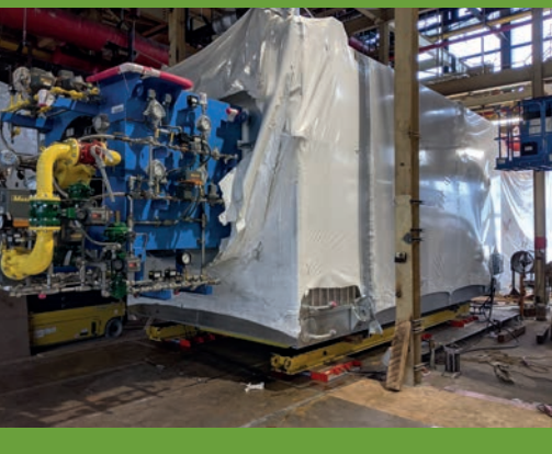
A skidding system was combined with air-skates on a lightweight “dance floor.”
