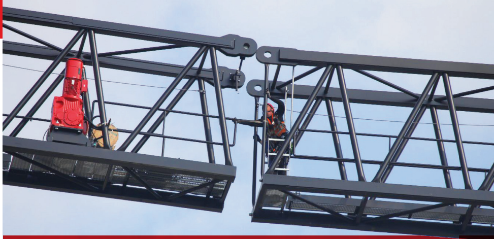
Fast jib section connection carried out by just one rigger
