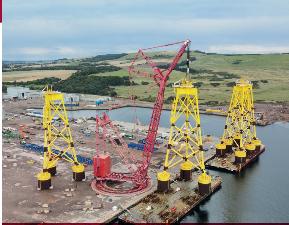
Mammoet worked at Nigg Energy Park near Inverness, Scotland, in separate phases to load-in, store, and load-out the turbine jackets, two at a time. Key to the project was the 3,200 tonne capacity class PTC 210 DS super heavy lift ring crane
