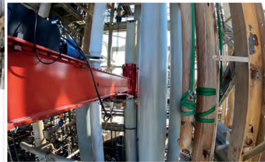
Barnhart utilized a moving counterweight cantilever beam to remove and replace 12 reactor legs.
