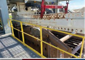
ProLift's solution involved two multipoint spreader bars fastened together forming a multi-point lifting frame, which was connected to ProLift's Bear Paw Cantilever System, which resulted in a Multi-Point Cantilever lifting frame.
