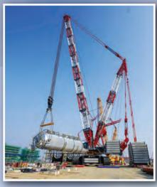
The water wash tower lift was executed within a highly congested refinery site, requiring exceptional precision in crane mobilization and load movement. A roundup of jobs that required highly specialized rigging equipment.
