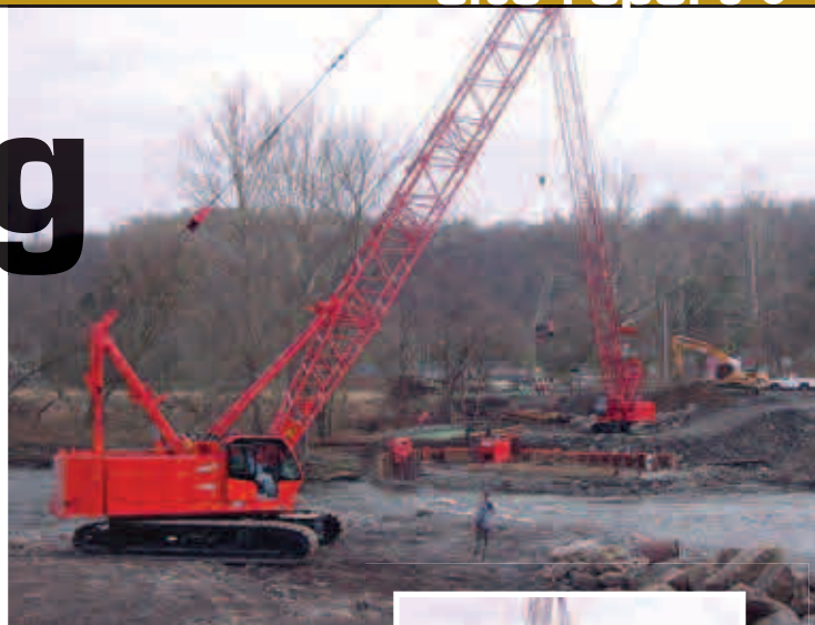
At times the two Model 10000 crawlers operate in tandem and other times independently on either side of the river. Their initial job was driving piles 90 to 100 feet deep
