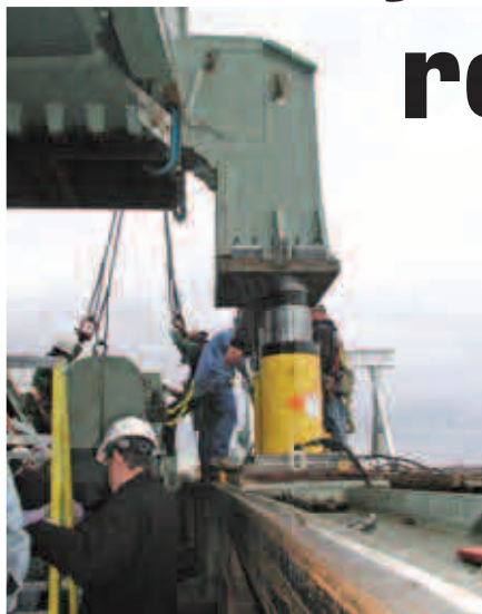
An old bogie being moved out. Two hydraulic Enerpac jacks are lifting against an add-on jacking bracket, as are another two jacks
