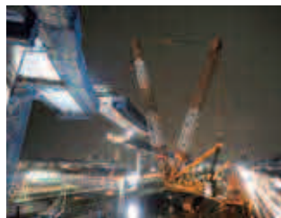
Two Kobelco crawlers install bridge beams overnight in Tokyo
