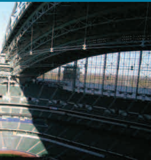
The retracted Miller Park roof – three roof panels are stacked on the right, two on the left
