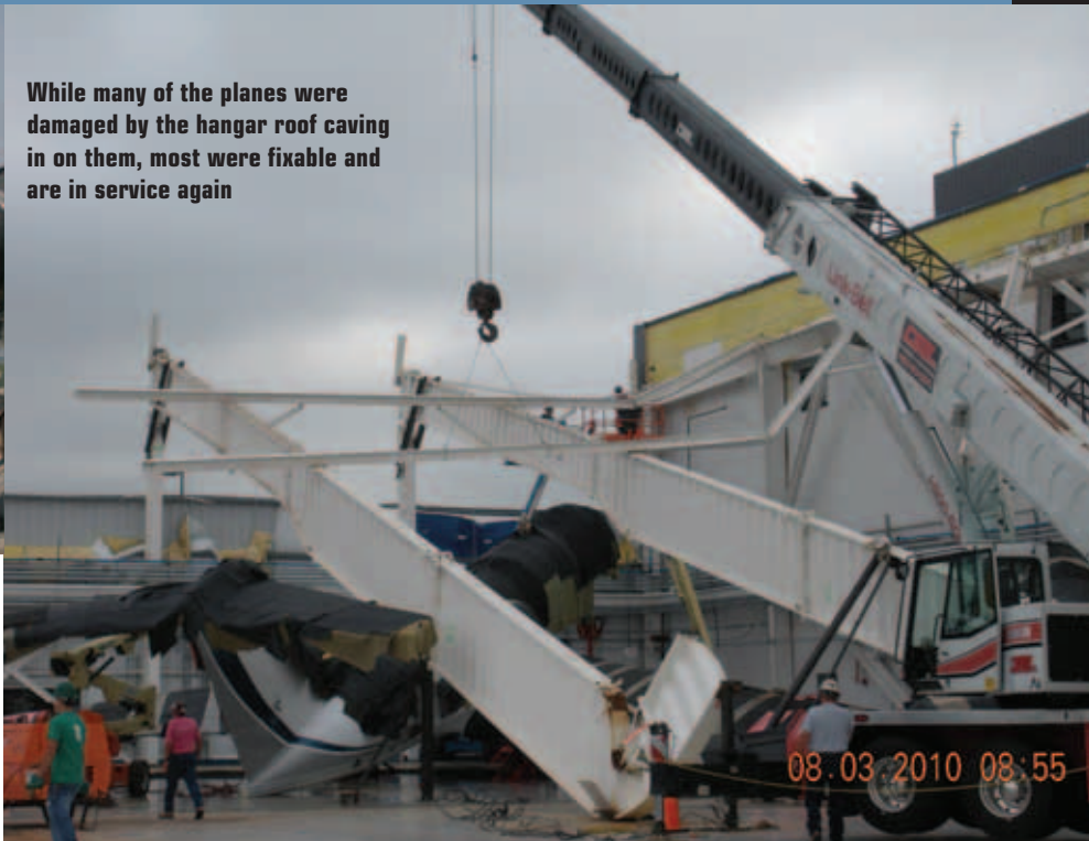
Among the most challenging lifts was the removal of the 165-foot-long girders that weighed 30,000 pounds each
