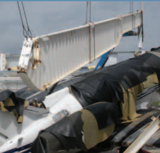
Among the most challenging lifts was the removal of the 165-foot-long girders that weighed 30,000 pounds each
