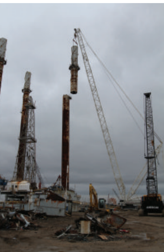
In Sabine Pass, TX, a Terex Demag 2800-1 makes modifications to drilling rig platforms
