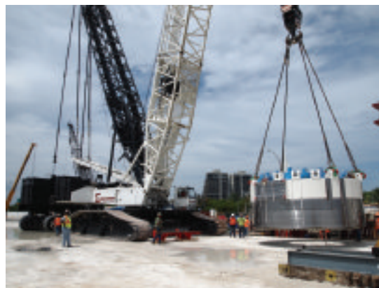
Buckner’s Liebherr LR-1750 lifts the drive motor section of the tunnel boring machine
