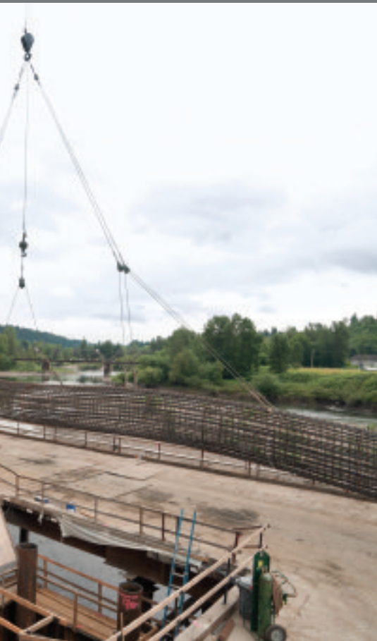
Hamilton Construction deployed its 110-ton 218 HSL on the I-84 Sandy River and Jordan Road Bridges project in Troutdale, OR. Equipped with 150 feet of boom, the 218 HSL placed 120-foot rebar cages
