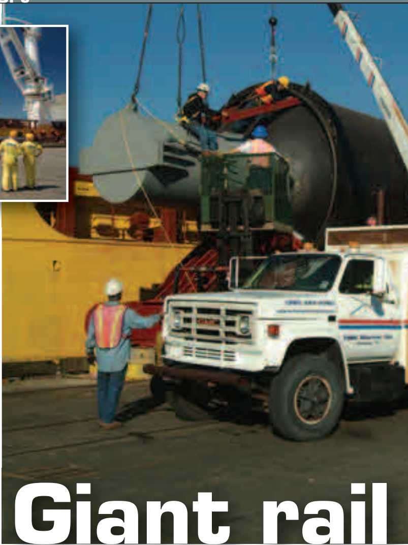
The 628 ton reactor being unloaded by Big Lift's Happy River on to Dock 16 in the Port of Houston
