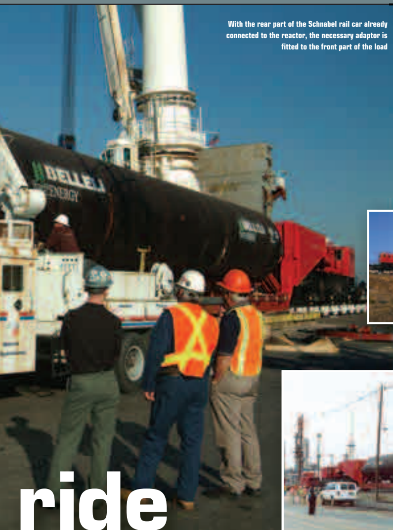
ABOVE: The reactor suspended between the Schnabels, or arms, of the 36 axle rail car combination
