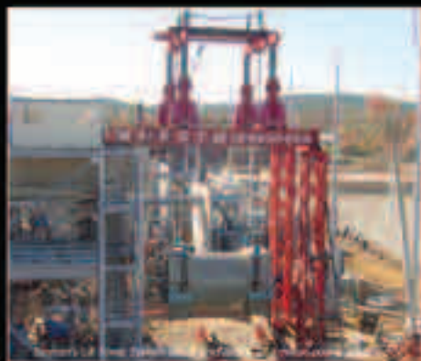
Emmert's Duty Beam Transporter—800,000 pound payload
