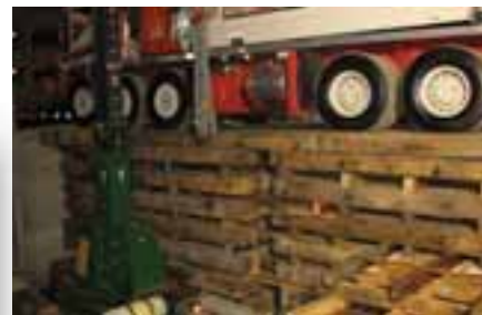
Olympic polyester slings rated at 200,000 pounds in a basket were attached to the outriggers of the crane and used to lift the machine 10 inches at a time
