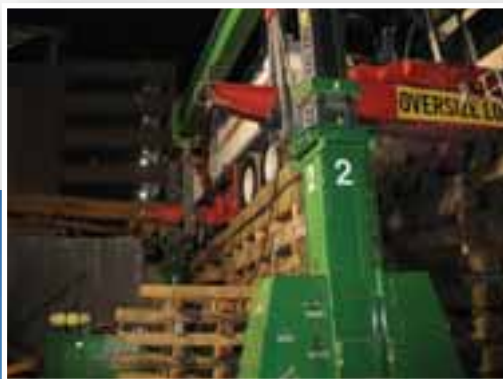
Olympic polyester slings rated at 200,000 pounds in a basket were attached to the outriggers of the crane and used to lift the machine 10 inches at a time
