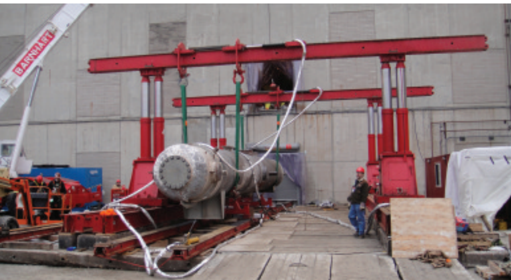
Barnhart Crane & Rigging used a Lift Systems gantry, slide track and 50-ton rough terrain crane to remove and replace three nuclear feedwater heaters
