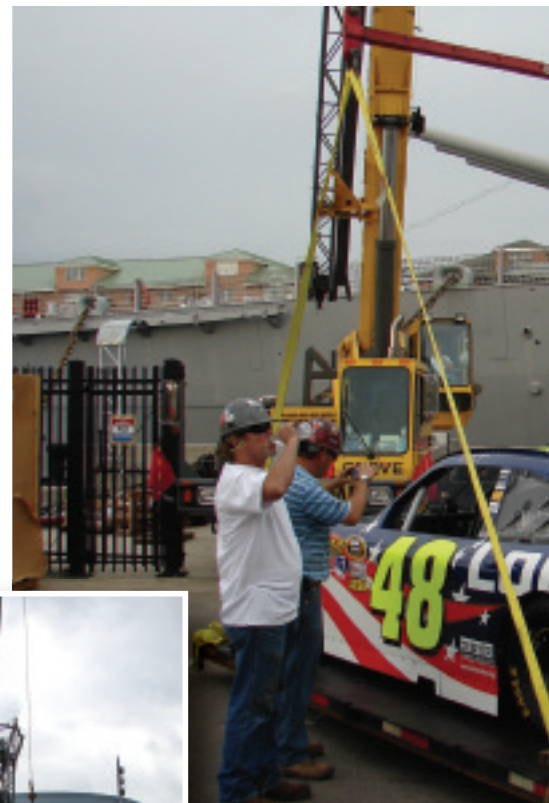
The Grove TMS 760E 60-ton hydraulic truck crane was rigged with 100 feet of boom at a radius of 45 feet
