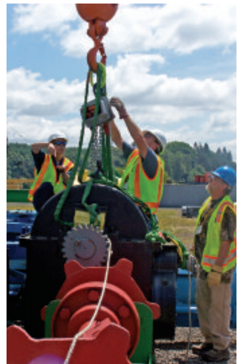
Using a chain hoist can help level the load
