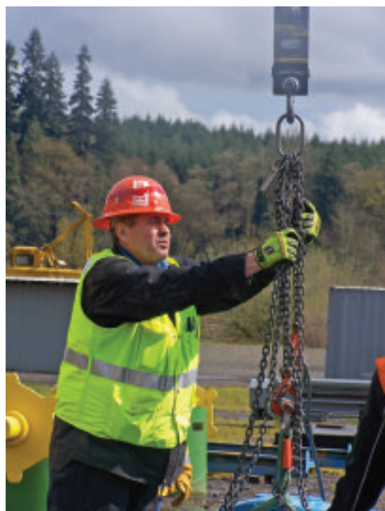
ABOVE: Straightening chain legs helps avoid link damage from twisting
