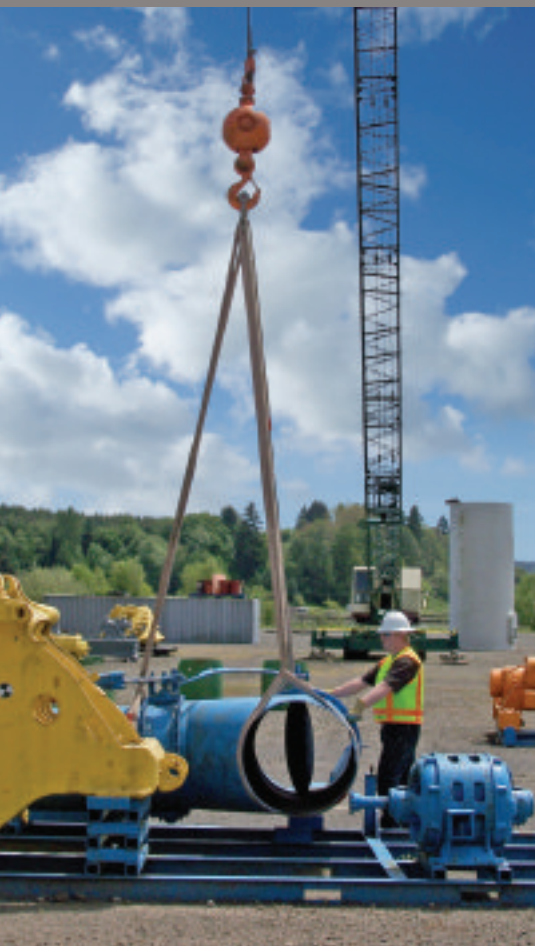
ABOVE: Rigging over the center of gravity will help keep the load level
