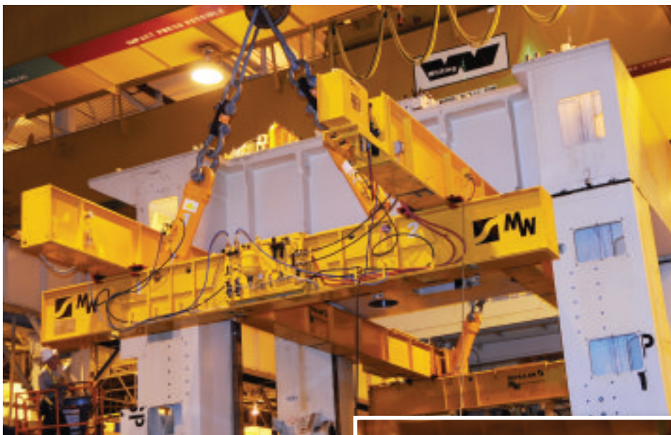
For a complicated press installation and restoration project, Schuler Mexico created the Flying Gantry
