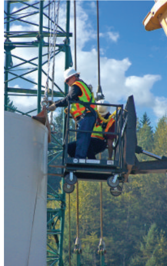
Braided wire rope slings and large shackles are used for a large lift
