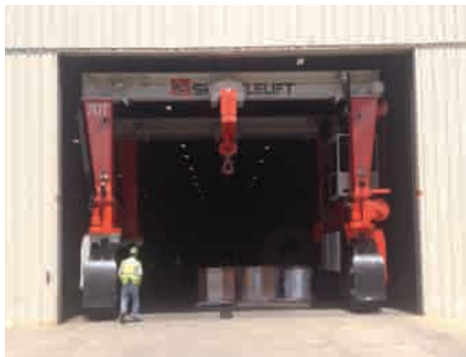
The Shuttlelift DB70 was designed short and stout so it could fit through Air Products' existing facility.
