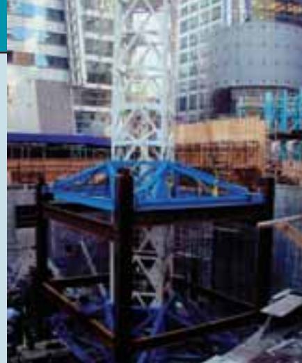
Steel erector Canron used a similar climbing device with an upper and lower basket (blue) for the Times Square Tower construction in New York. Note the sliding foot members at their outriggers
