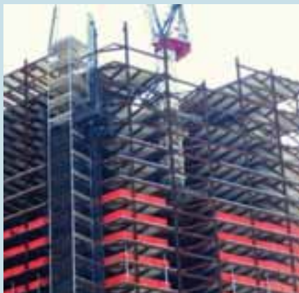
Falcon Steel adapted the TG tower crane external climbing cage for internal climbing by adding a jumping frame and upper support beams, both grey and equipped with extendable outriggers
