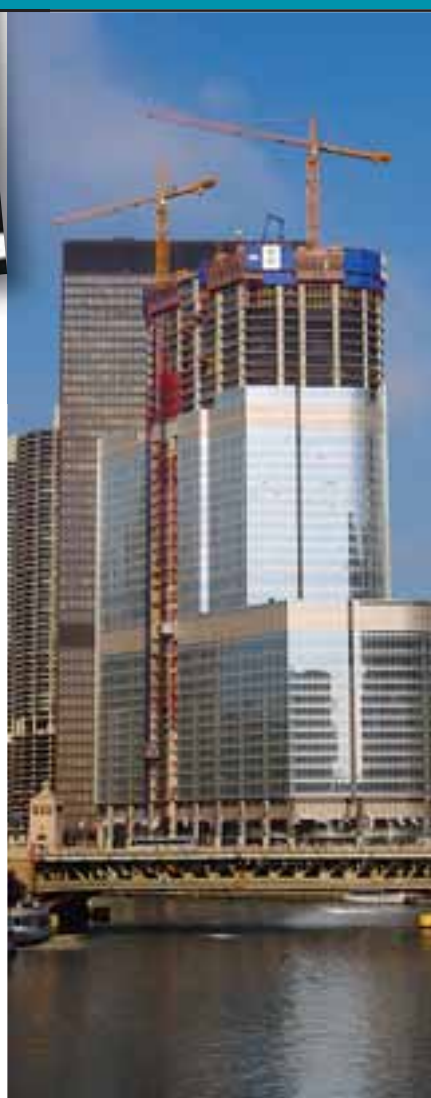
Supplied by Morrow, two Liebherr 420 EC-H 16 Litronic cranes work on the Trump International Tower and Hotel in Chicago. Contractor is James McHugh Construction. Full hook height will top 1,100 feet
