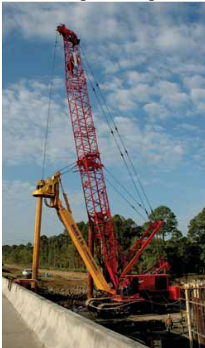
A barge-mounted Manitowoc Model 1015 is drilling shaft foundations in Georgia
