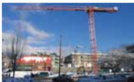
A Wilbert WT 200 e.tronic with shortened jib working on a poured concrete mid-rise project in North Vancouver, British Columbia
