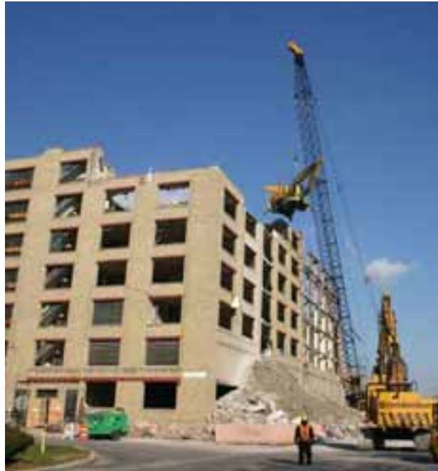
A 150-ton Liebherr crawler crane lifts a demolition excavator to the top of a building
