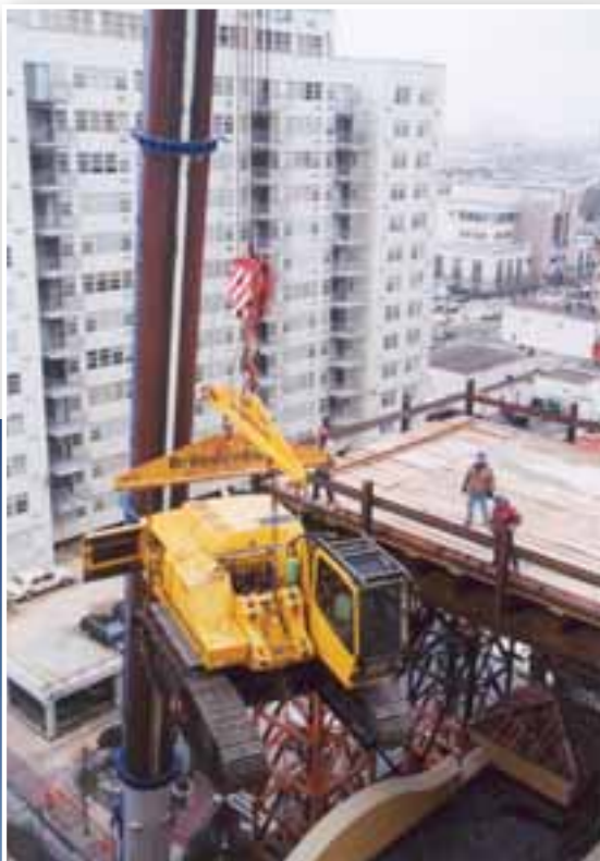
A 500-ton truck crane places an excavator on top of a building slated for tear-down
