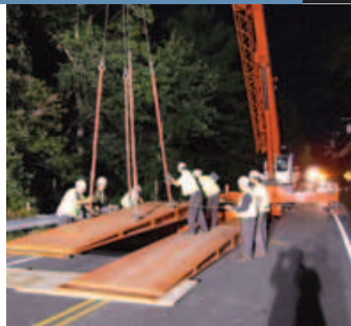
A 45-ton truck crane was needed to set the decking and wedges required for the bridge jumping system. The crane travelled with the convoy throughout the journey
