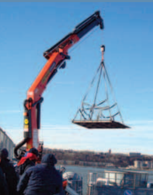
The Palfinger PK 150002G with PJ 170E jib lifts materials to be used for the installation of the smaller Palfinger crane as well as its power unit, shown in the foreground
