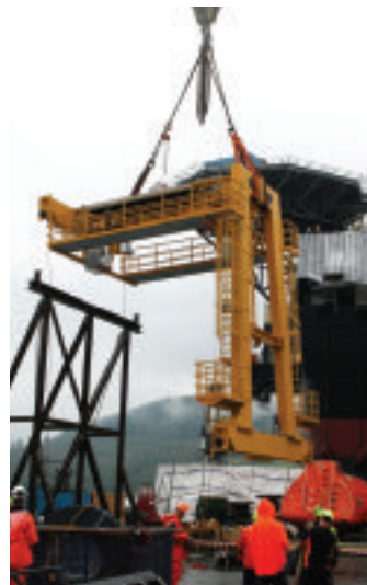
The A-frame and track beams were assembled in Norway before the crane system was transported to the rig
