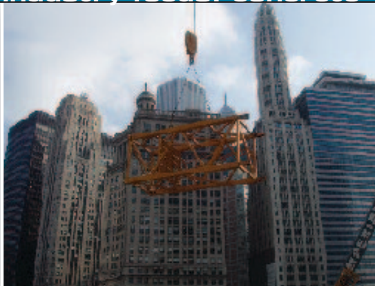
A Liebherr 420 ECH tower crane helps to erect another Liebherr 420 ECH tower crane at the site
