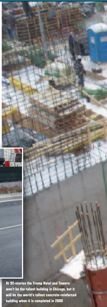
Dale Hendrix, executive vice president of McHugh Construction, oversaw The Big Pour which involved the continual pouring of 5,000 cubic yards of concrete into a "mat hole," which would form the underground foundation for the concrete reinforced building
