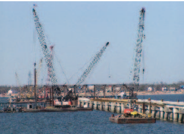
Crews are working 24-7 to fix CSX railroad bridges washed away by Hurricane Katrina
