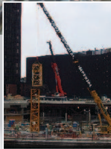
The Liebherr 420 ECH picks up the tower crane sections off the truck and swings them around to a staging area on the ground. At that point, a 175 ton Krupp all terrain crane owned by Imperial Crane lifts the section upright and then swings it over to the base of the tower being erected. Crews catch the section and secure it to the base
