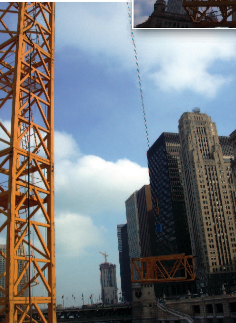
A Liebherr 420 ECH tower crane helps to erect another Liebherr 420 ECH tower crane at the site
