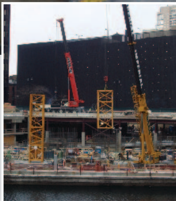
The Liebherr 420 ECH picks up the tower crane sections off the truck and swings them around to a staging area on the ground. At that point, a 175 ton Krupp all terrain crane owned by Imperial Crane lifts the section upright and then swings it over to the base of the tower being erected. Crews catch the section and secure it to the base
