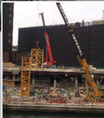
The Liebherr 420 ECH picks up the tower crane sections off the truck and swings them around to a staging area on the ground. At that point, a 175 ton Krupp all terrain crane owned by Imperial Crane lifts the section upright and then swings it over to the base of the tower being erected. Crews catch the section and secure it to the base
