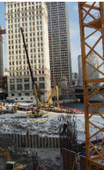
Dale Hendrix, executive vice president of McHugh Construction, oversaw The Big Pour which involved the continual pouring of 5,000 cubic yards of concrete into a "mat hole," which would form the underground foundation for the concrete reinforced building
