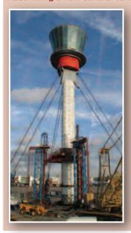
The recent expansion of London's Heathrow Airport necessitated a new control tower. The lifting and transportation contractor (Fagioli PSC Limited, Iver, Buckinghamshire, United Kingdom) worked with the steelwork contractor (Watson Steel, Bolton, Lancashire, United Kingdom) to minimize disruption and keep construction equipment below the radar ceiling so that airport operations could continue safely.
