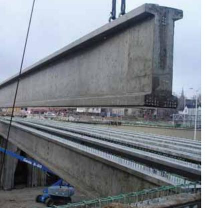
"The major work has been the demolition work and also setting 147,000 pound bridge beams," he says. "We've been setting these beams with two cranes, a 110 ton capacity Terex and the Manitowoc 4000. It takes two crane picks, simultaneously."
