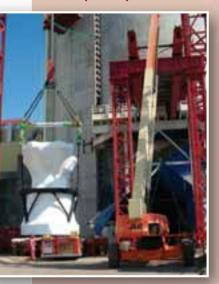
The Steam Generating Team Ltd, Charlotte, NC, called on Mammoet USA, Rosharon TX, to help replace a reactor head weighing 172,674 pounds and two steam generators weighing 1,144,500 pounds each at a nuclear power plant in Russelville, AR. Judging the lifting equipment already inside the containment building to be inadequate
