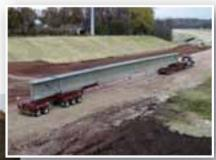
Span Crete Inc. fabricates the girders used on the Marquette Interchange. The company hauls the girders, which range from 60 to 140 feet long, using a 48 foot lowboy with a bunk on it and behind that a four axle steerable unit
