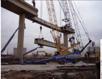
A 150 ton capacity Liebherr and a 215 ton capacity Terex assist in demolition, slowly bringing down a section of the old bridge span
