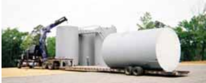
Setting tanks with the Autogru PM model 47025P knuckle boom crane
