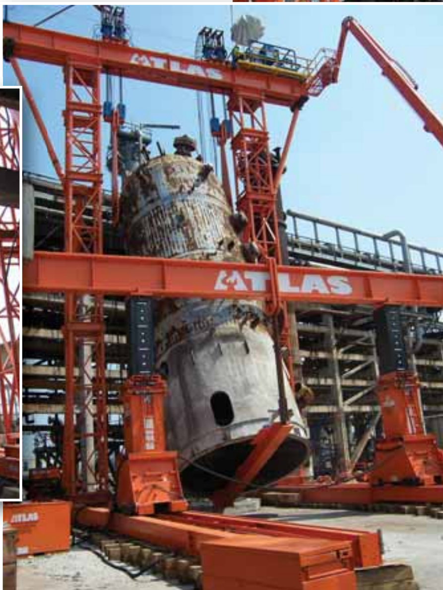
The tower sections and header beam assemblies would be rigged to rise to more than 70 feet top elevation
