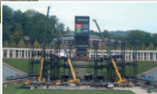
Two Grove TMS760E truck cranes being used last year to erect a stage for a Rolling Stones concert in Virginia
