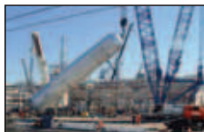
Hoisting 400 Ton Vessel
