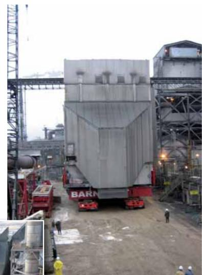
Out of the box thinking was required to replace a boiler in a forest products company mill while at the same time keeping the mill online Barnhart team worked around the clock to jack, slide, lower, transport and re-erect the 600-ton ESP box. The job featured many unique tools such as the custom integrated jacking system, a 1,000 ton slide system, the Barnhart Modular Lift Tower and new Goldhofer PSTe electronic steer trailer. Each move was completed ahead of schedule in only 11 days.
