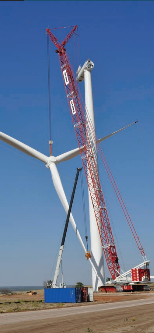
KR Wind's Terex Demag CC2800 is the main crane on a wind farm in Oklahoma
