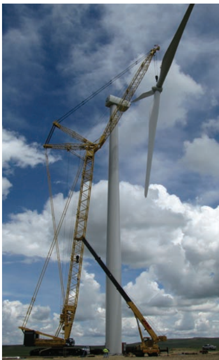
KR Wind's Terex Demag CC2800 is the main crane on a wind farm in Oklahoma
