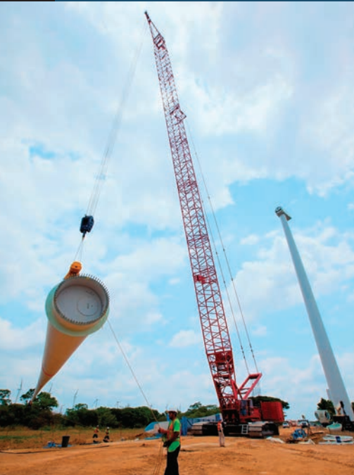
A Manitowoc 16000 fitted with a wind attachment erected 204 turbine towers on a wind farm at La Ventosa, in the Juchitán district of Mexico's southern state of Oaxaca
