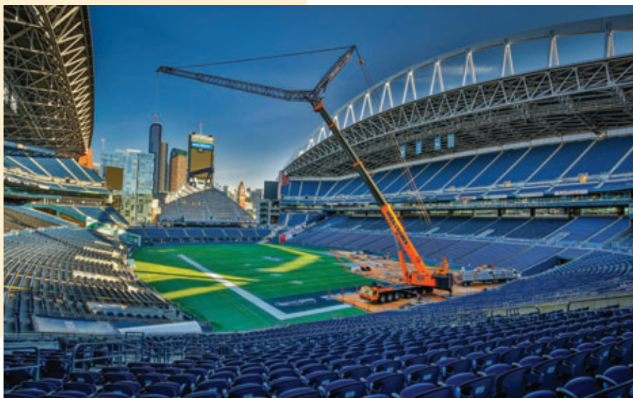
PHOTO: Ness & Campbell Cranes
