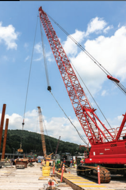
The Manitowoc 11000-1 was chosen because of its versatility in setup. It was erected on a trestle, which has a steel platform with wood on top to support the crane.
