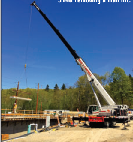
Ness & Campbell's HTC-3140 removing a man lift.
