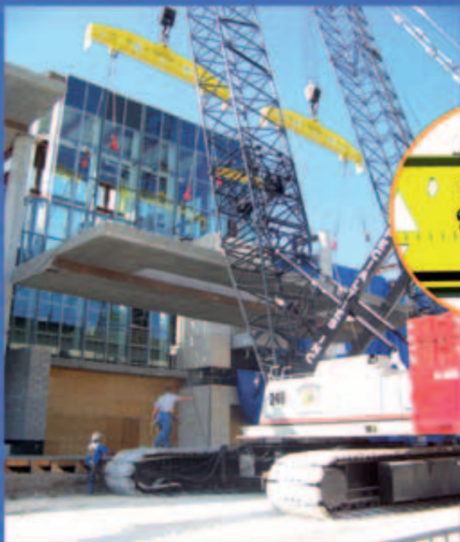
Two Super-Bars Hold a 339,000 Pound Wall.
