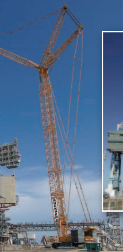
New weather protection doors, which protect the shuttle during the time it is mounted at the launch pad prior to the launch, were installed on a sliding trolley. The 52,000 pound doors were lifted at a 120 foot radius
