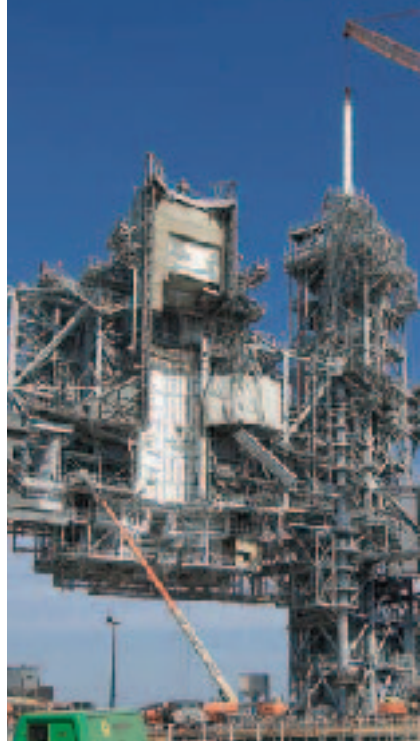
Resembling a big pipe, the 47,000 pound candlestick is fixed above the launch pad structure. Buckner's new Liebherr LR 1400/2 lifted the device to a height of 365 feet at a 140 foot radius
