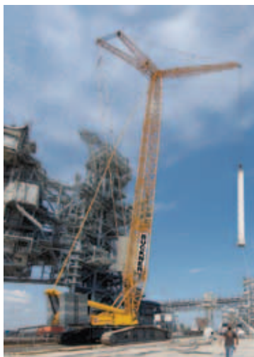
The tallest point on the launch pad, the "candlestick" is designed to attract lightning from as far away as five miles, protecting the Space Shuttle and its sensitive electronics from lightning strikes
