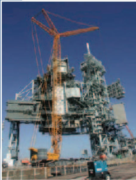
New weather protection doors, which protect the shuttle during the time it is mounted at the launch pad prior to the launch, were installed on a sliding trolley. The 52,000 pound doors were lifted at a 120 foot radius
