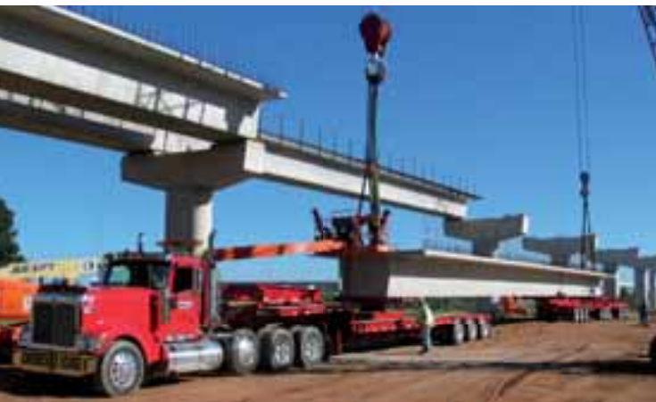
The 104 girders vary from 40 to 140 feet in length with widths ranging from 12 to 16 feet. They weigh from 40 to just over 100 tons
