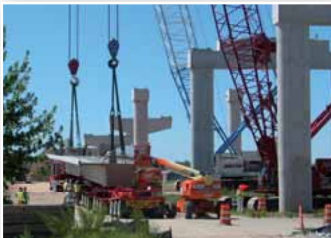
The ERM nine-axle Hydra-Steer trailer with dual steering enhances the load and go skid steer method with new single frame steering capability. The steering improves the versatility during extremely heavy loads and back hauling
