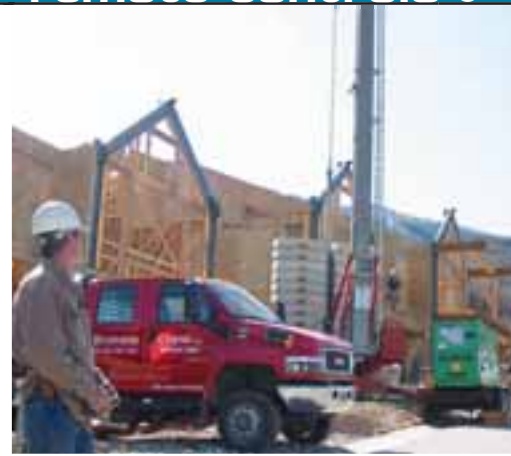
Earl Bronson operating a NBB model Nano 2S controller running a Comedil CBR-32 self erecting tower crane at the Star Mountain Construction job site in Park City, UT
