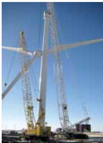
Wanzek Construction's Demag CC-2500-1 (550-ton) and Kobelco CK1000 (100-ton) installing rotor on wind tower at the Endeavor Wind Farm near Harris, Iowa
