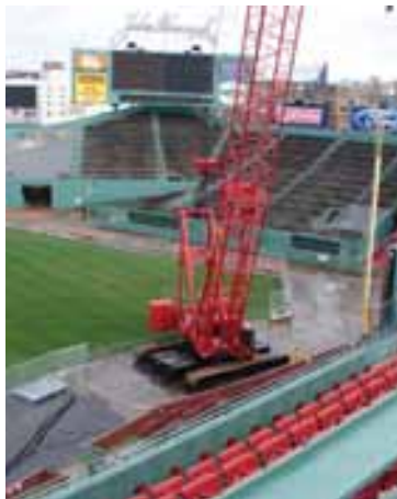
Crane operator Mike Morgan had his work cut out for him, especially when removing and replacing the large light poles from the construction area. Booming out 170 feet, he handled the 35,500-pound poles with ease
