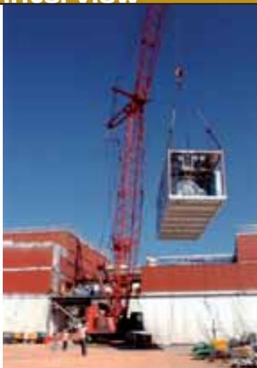
Southern handled the erection and interconnection of a modular pharmaceutical plant in Durham, NC
