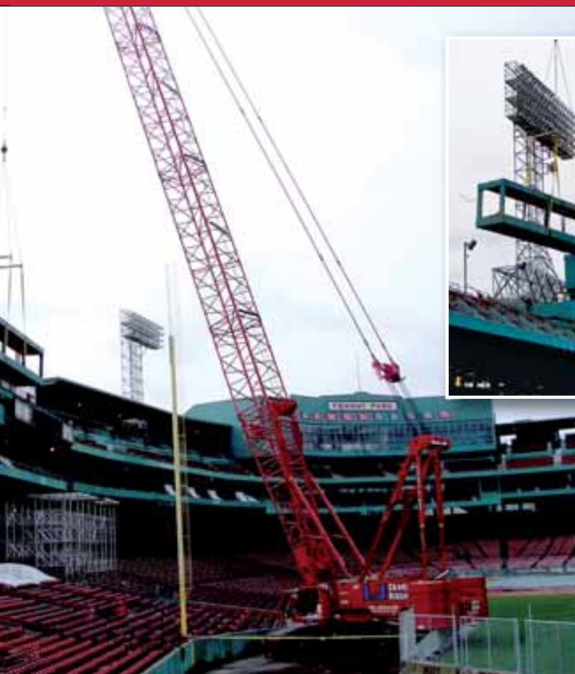
The cranes were partially disassembled and brought into the ballpark via the "Green Monster"
