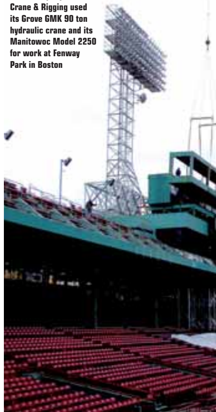
Crane operator Mike Morgan had his work cut out for him, especially when removing and replacing the large light poles from the construction area. Booming out 170 feet, he handled the 35,500-pound poles with ease
