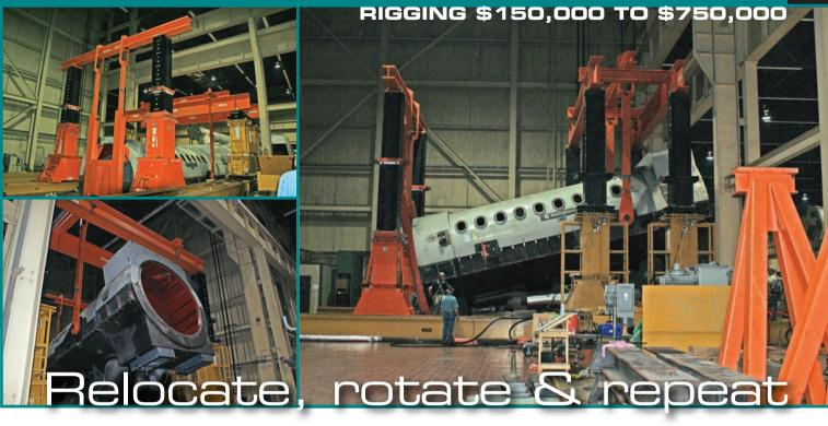
n January 2011, at the peak of the winter lighting and heating season in Ohio, a generator at FirstEnergy Corporation's Sammis Station threw its rotor. National Electric Coil (NEC) was dispatched to perform the emergency repairs. NEC in turn called Columbus, OH-based Atlas Industrial Contractors to assist in the tedious job of rebuilding the damaged generator.
