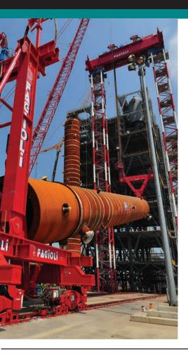
14-feet high. Equipment used on the job included a high girder bridge adapted to a pair of modular platforms with 10 hydraulic lines each. Absolute accurate planning was required to avoid disruption of rural villages in very poor condition and several bridges unprepared for a heavy load.
