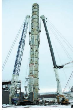
Once the tower was freed from its base, the two cranes worked in tandem, sharing the load. There were still a few unknowns, such as the major weight of the reconditioning tower
