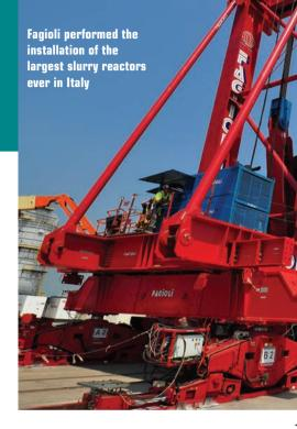
jacks, four skid shoes, an 80-meter high tower lift system utilizing four L600 strand jacks and a swivel system. Before the operation, Fagioli performed a test load of 2,400 tons in order to guarantee maximum safety.
