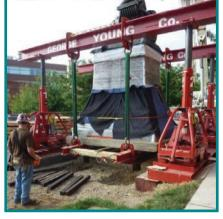
Prior to handling and rigging the monument, the granite's multiple fissures were injected with epoxy to stabilize the stone. Areas where engraved lettering was unstable were fortified with Japanese Tissue, a long-fiber vegetable material. Corners were edged in protective devices, and Ethafoam was placed between the rigging equipment and the monument base to absorb vibrations that might cause fissures to spread.
