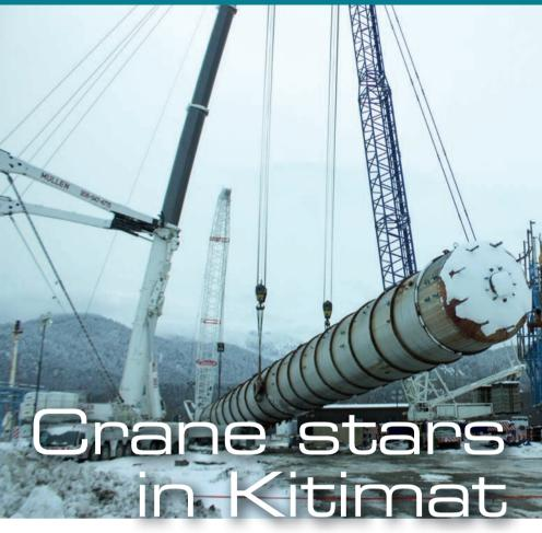
Onsite were the two largest cranes in Northern's fleet, a 1,350-ton capacity Liebherr LTM 11200 and a 1,000-ton capacity Liebherr LG 1550, according to Pat Carrigan, director of sales and marketing for NC Services Group Ltd., Northern Crane's parent company.
