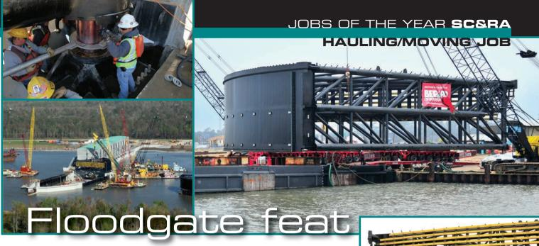
erard Transportation, Inc., based in Loreauville, LA., provided transportation and rigging services to move the world's largest flood sector gates from the fabricator's vard in Houston to the final operating position in waters south of New Orleans, LA. Each of the two 690ton floodgates measured 130-feet long by 120-feet wide by 32-feet high.
