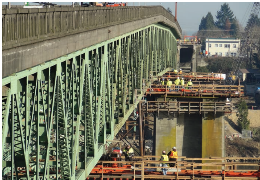
Omega Morgan crews moved the old Sellwood Bridge to a temporary location until the new bridge can be constructed.
