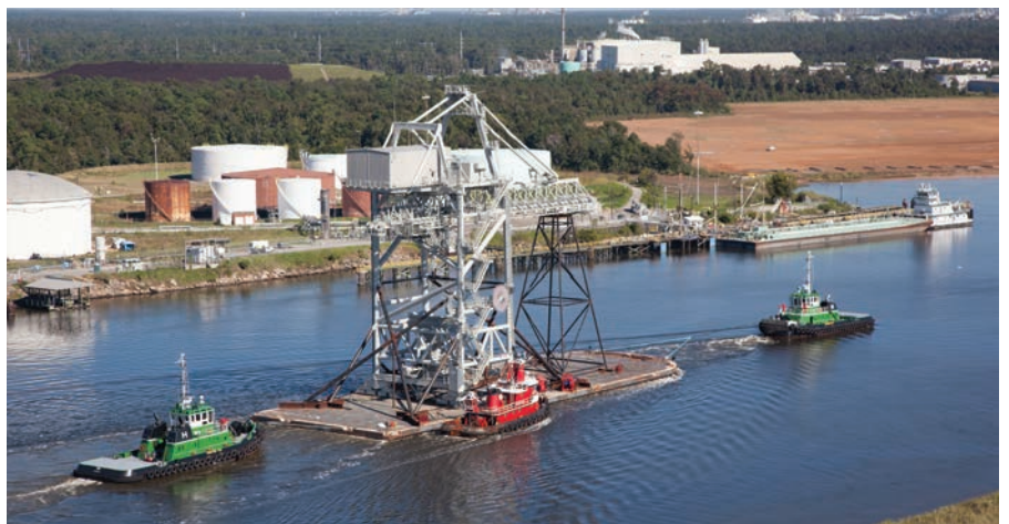
Transporting and installing a giant ship unloader crane required precision planning by Berard Transportation.
