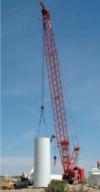
With ease a Manitowoc 999 owned by Buckner HeavyLift sets in place the lower portion of a wind turbine
