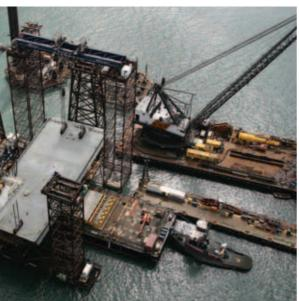
Each tub was lifted from a barge used for transport from Portland, OR, where they were fabricated. As with first span, a temporary support tower has been skid under the span to hold it in place for three months until the concrete joint with the existing Skyway is poured and cured, filling a gap of some 6 feet. The San Francisco (west) end of the tub is being supported by another temporary tower until the suspension bridge is constructed.
