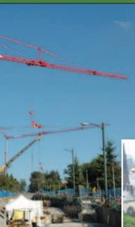
LEFT: Five Potain self erecting tower cranes are working on a \$1.7 billion rapid transit project in Vancouver, BC. Portions of the rail line will be underground. Rather than drill a tunnel, contractors chose a cut and cover process where the self erectors follow the trench to build walls
