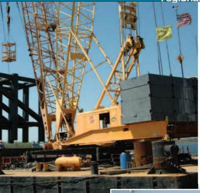
Left: Several Manitowoc 4100 Ringer cranes have worked from barges repairing the damaged levee system in New Orleans. Initially the cranes were removing debris washed into the waterways. Today they install massive flood wall storm gates
