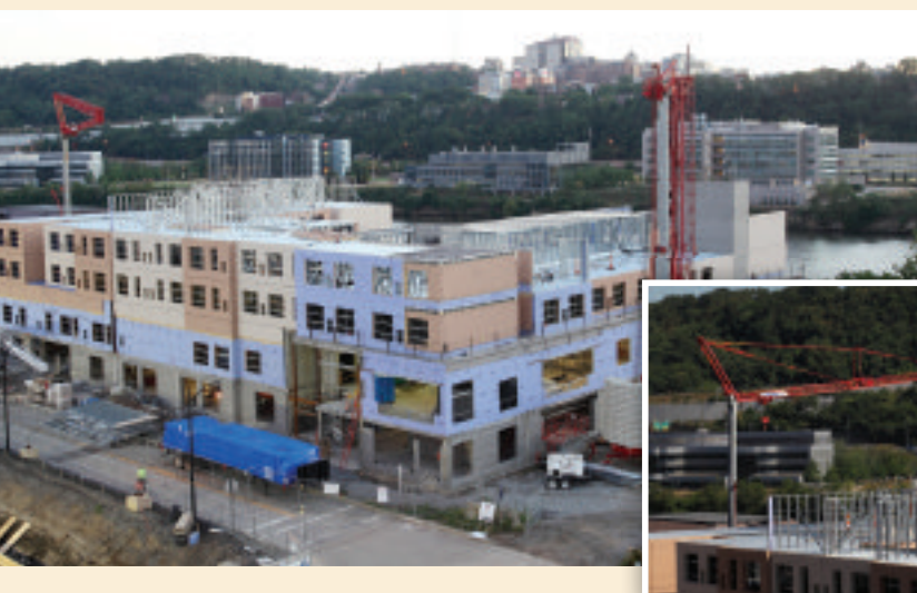
A Potain Igo 50 and Potain HDT 80 work on a hotel construction site in Pittsburgh, PA
