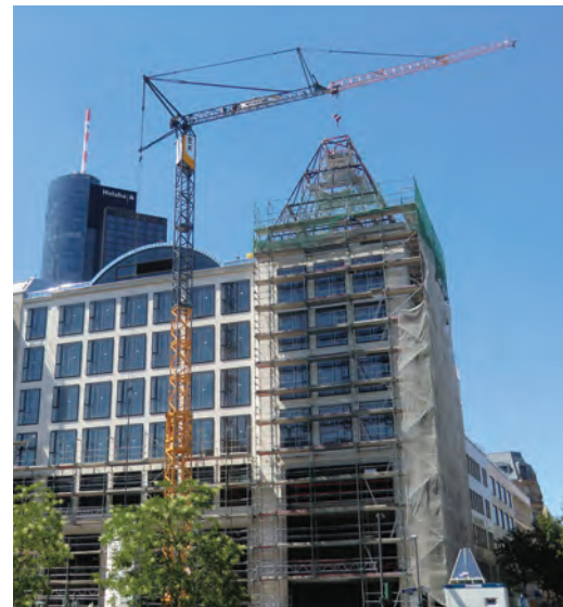
Liebherr's 81 K, pictured here in Frankfurt, Germany, is the most popular self-erector, the company says.
