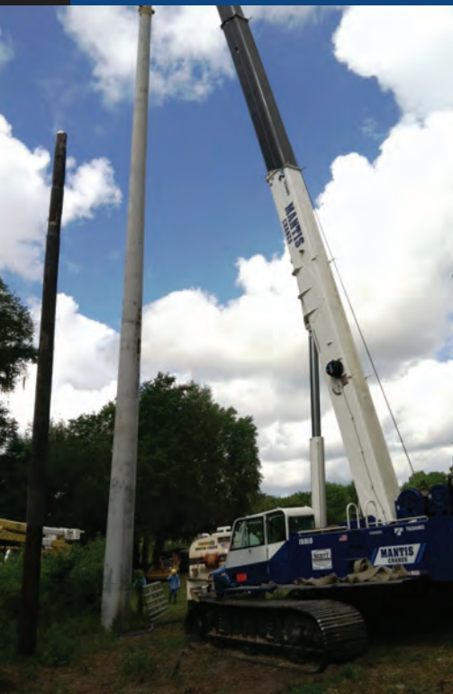
The Tadano Mantis telescopic crawler has the flexibility of operating in more challenging terrains and environments.
