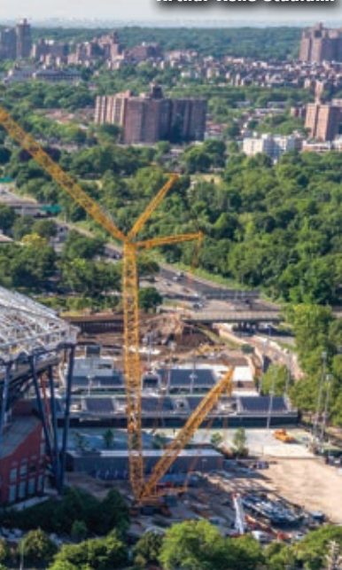
Three Buckner HeavyLift crawlers install a retractable roof on the Arthur Ashe Stadium.
