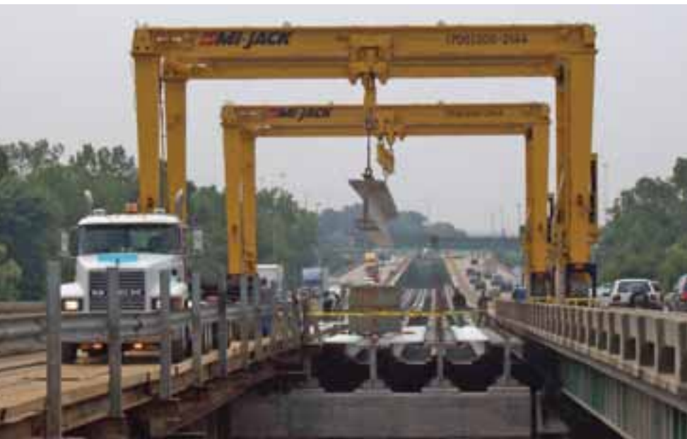
A Mi-Jack Travelift gantry crane was an asset in a bridge building effort in Alabama
