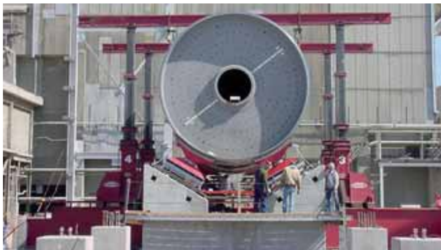
A J&R Engineering 450-ton capacity gantry is used to place a ball mill into its journals after receiving it from the transporter
