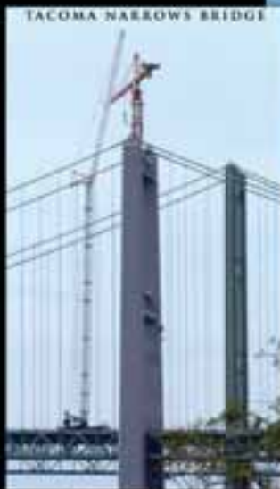
TACOMA NARROWS BRIDGE DEMAG - TC1200 472' ROOM
