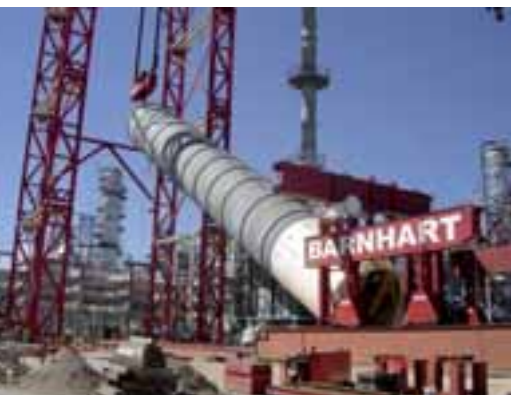
Lift Systems 48A gantry in position after transferring the "tail" of a 900-ton reactor from the transporter to the Barnhart Modular Tailing Tower (MTT)
