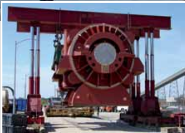
A Lift Systems 48A gantry transfers a 350-ton generator to a transporter for on-site movement to the erection area
