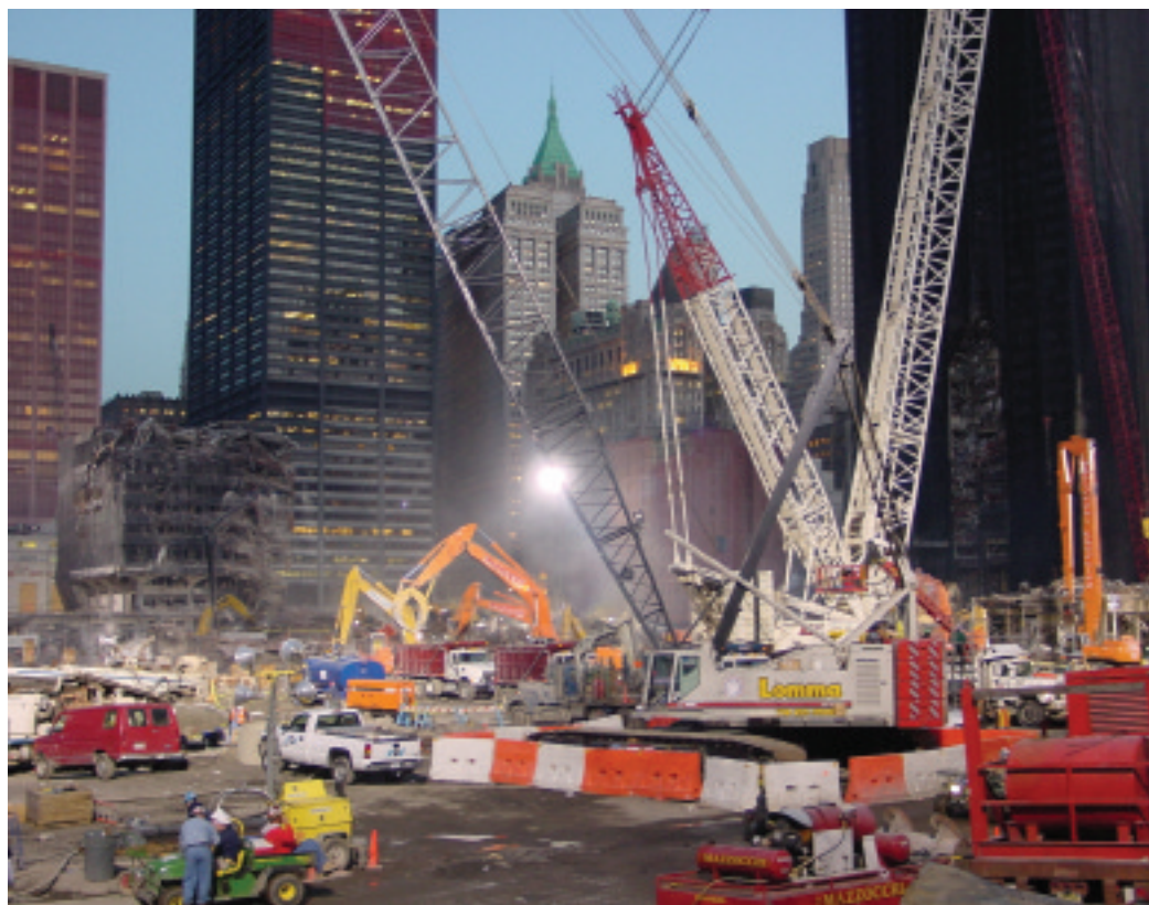
Ground Zero was divided into four quadrants. As many as seven cranes were operating in each quadrant, lifting steel and removing rubble
