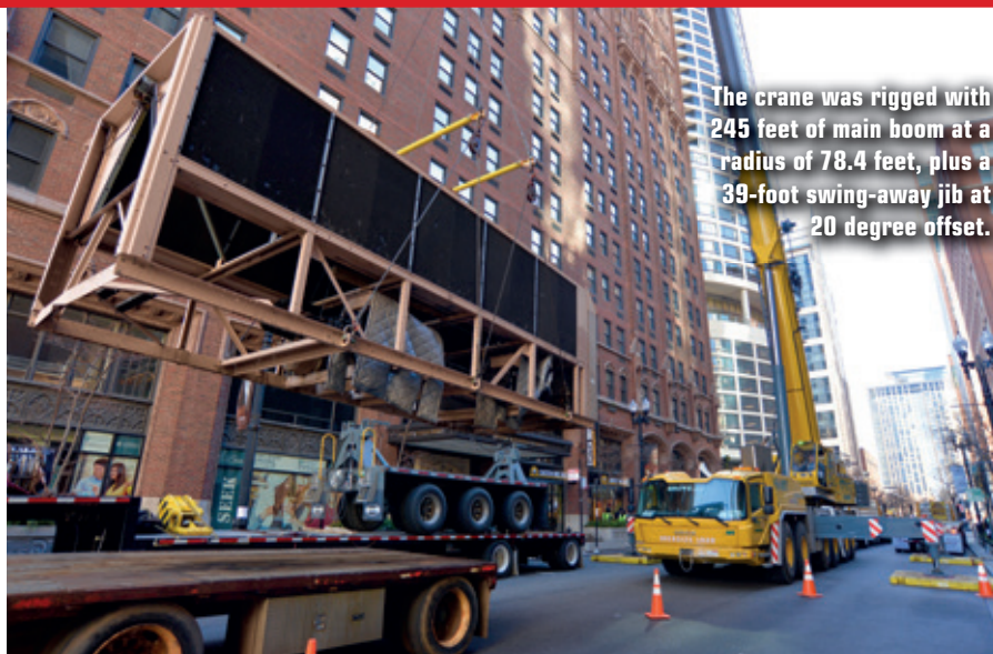
The GMK 6300L was rigged with its full counterweight of 220,000 pounds. Fully rigged the crane was set up at 38-foot wide including the outrigger mats setting up on a 40-foot wide street.
