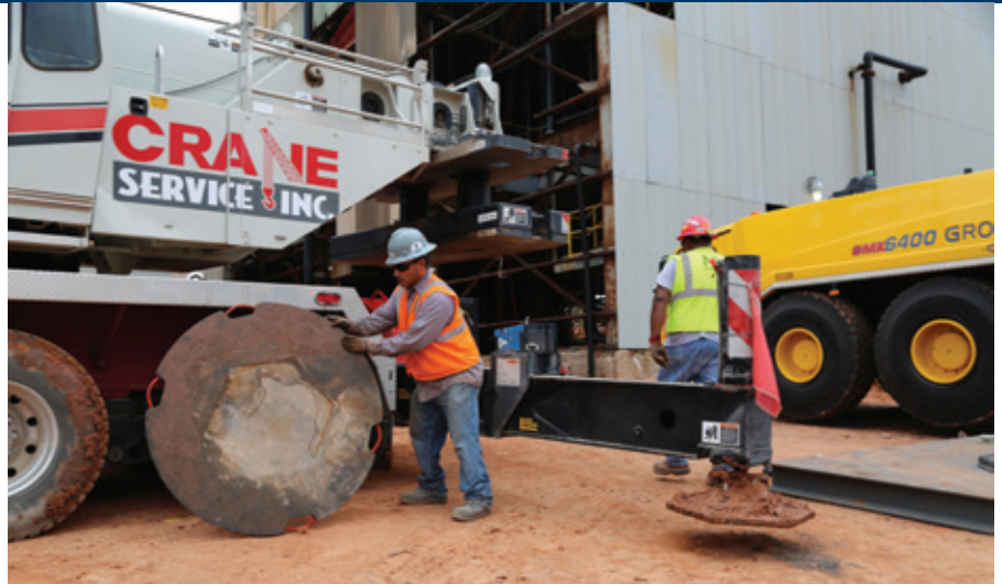
Round outrigger pads are easier to roll into place.
