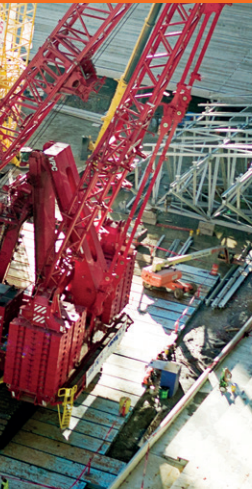
Maxim CraneWorks' Manitowoc 31000, with a capacity of 2,535 tons, recently finished installing the complicated roof system at the new Atlanta Falcons stadium.
