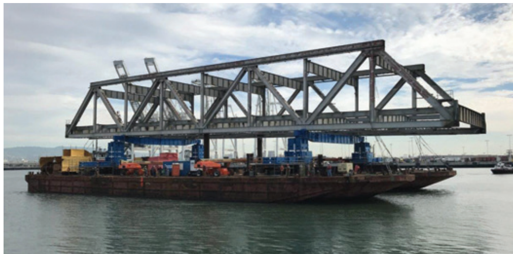
Utilizing its BPU-750 jack-up system stationed on top of a pair of 250 by 72-foot barges, Burkhalter removed spans from the old San Francisco-Oakland Bay Bridge.
