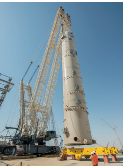
A Demag CC 8800-1 TWIN, with a capacity of 3,200 tons, works at a refinery in Qatar.
