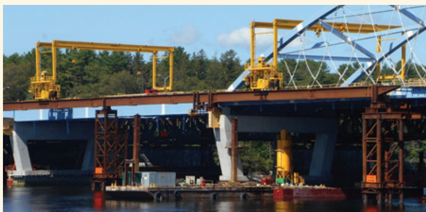
Two Mi-Jack MJ85s gantries were built with bogey-style rail wheels, a 103-foot inside clear width and a 40-foot hook height. The job required the machines to be 'launched' with the structures as the bridge was built over the river.
