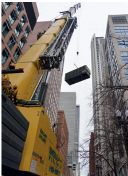
It was critical that the crane be in the exact right position. The lift plan was an important element and assured the clearances and safety factors were met.
