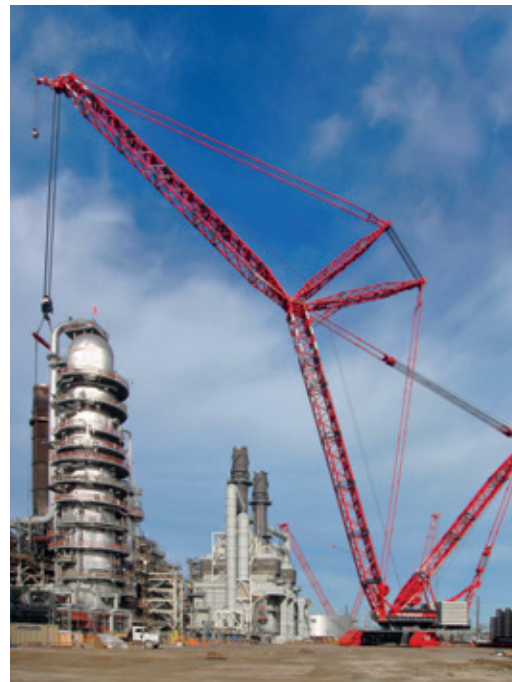
At 3,300-tons capacity, the Liebherr LR 13000 is the largest conventional crawler crane in the world. The first LR 13000 to work in the United States was in 2013-2014 at the Whiting Refinery in Illinois.
