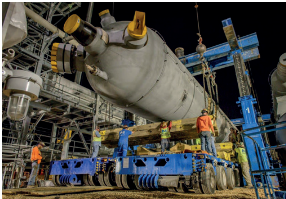
Burkhalter used two J&R Engineering 500-ton gantry systems to lift a 1.8 million-pound converter.
