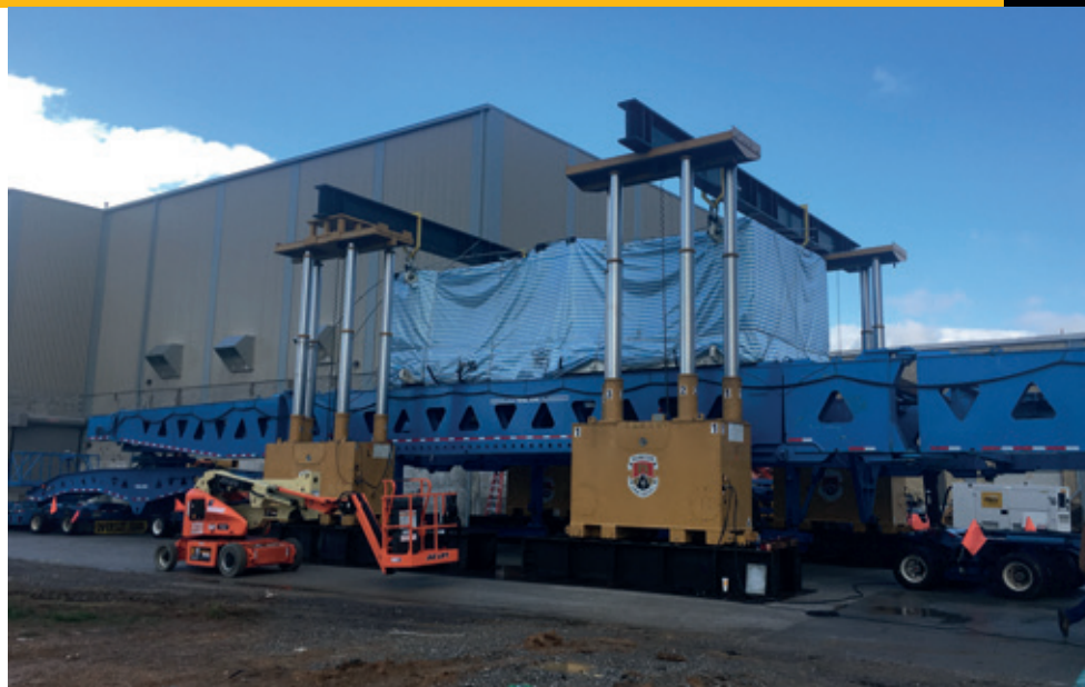
Two 600 ton E-Z Lifter gantries are being used in an ongoing gantry project unloading a variety of stamping press components in Georgia and Tennessee.
