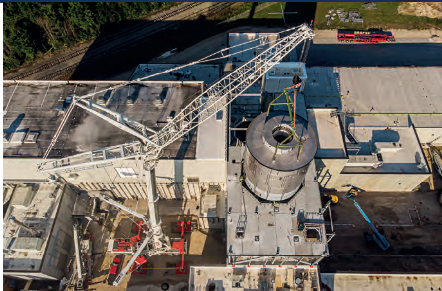
The 600-ton Liebherr LTM 1500-8.1 with VarioBase allowed the machine to move in closer.
