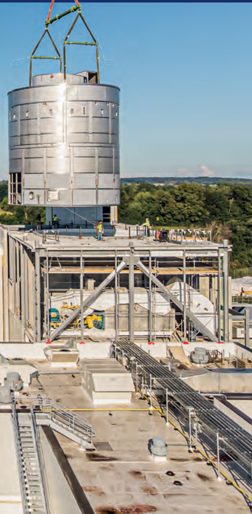
The 600-ton Liebherr LTM 1500-8.1 with VarioBase allowed the machine to move in closer.
