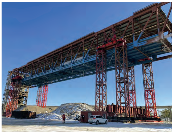
The 2,480-ton, 440-foot main truss of the Joe Louis Arena was lowered from an elevation of 82 feet to 20 feet.
