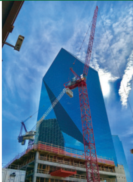
The $289 million Louisville Omni Hotel is being built with the assistance of a Terex SK575 tower crane and two Terex SK415 units on rent from Maxim CraneWorks.
