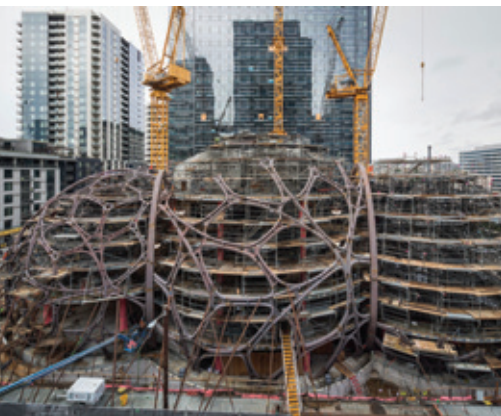
Morrow Equipment provided three Liebherr tower cranes to erect the Seattle Biospheres.
