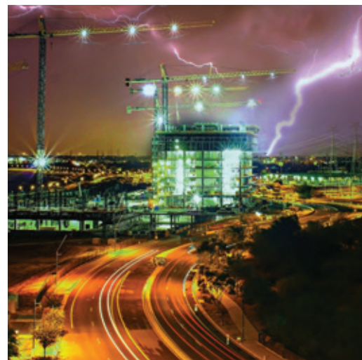
Five Terex Peiner SK-575s assisted in the construction of five State Farm office buildings that now stand overlooking Tempe Town Lake.
