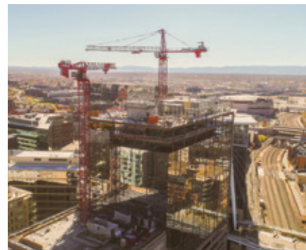
GE Johnson Construction awarded the contract to RMS Cranes for a 22-ton capacity Potain MD 485B tower crane on The Coloradan
