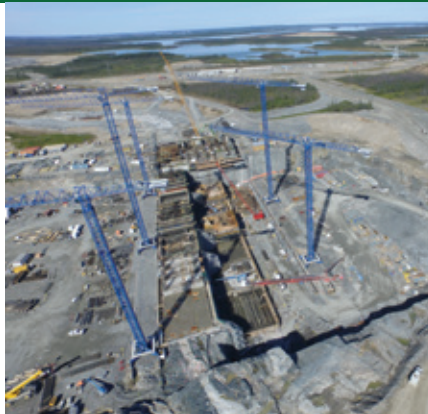
Five Linden Comansa tower cranes are working on the Keeyask Hydro Dam project in Manitoba, Canada
