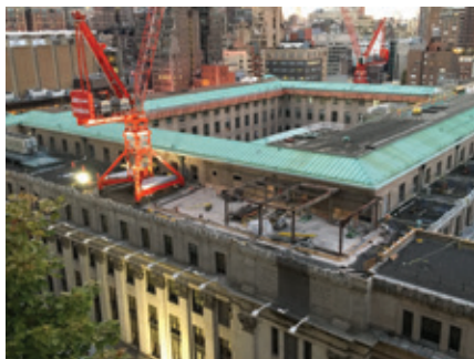
JK Crane, working in partnership with Skanska USA, provided two Potain MR-295s to work on the Moynihan Station project in New York City.
