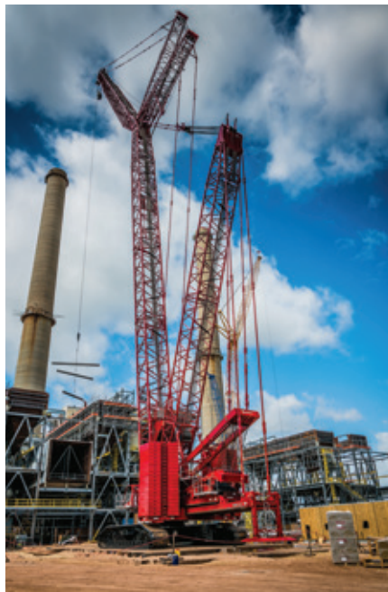
The biggest lift so far has been a 101-ton segment of duct work, which the MLC650 lifted to a height of 211 feet.
