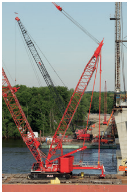
Kraemer North America is using a Manitowoc MLC300 to help replace the 2,482 foot-long Savanna-Sabula Bridge near Savanna, IL. The crane is erected on a 70 by 195-foot a barge in the Mississippi River, and it is lifting 76-ton arch rib sections to a height of 165 feet.
