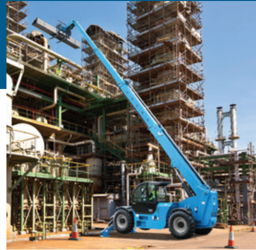
An overwhelming majority of crane operators believe that operators of telehandlers (such as the one pictured) should have to be certified.
