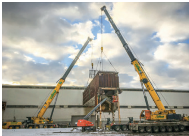
The demolition project took around 15 hours of work to complete.
