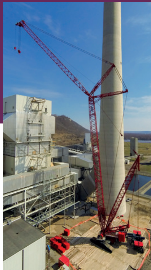
TNT Crane & Rigging's Liebherr LR1600/2 works in Wisconsin at Dairyland Power.
