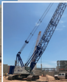
Bigge Crane & Rigging's 160-ton capacity Kobelco CK1600G works at a multi-billion dollar Liquefied Natural Gas Pretreatment facility in Freeport, TX. The crane is erecting steel sections that weigh up to 10,000 pounds each.
