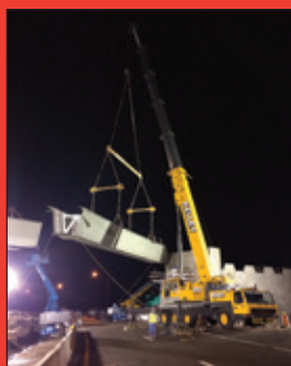
240 Ton Setting Tub Girder
