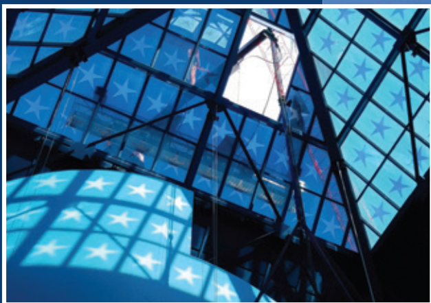
The counterbalance beam is visible through the glass and at the 8 by 8-foot opening. The working platform can be seen through the glass.
