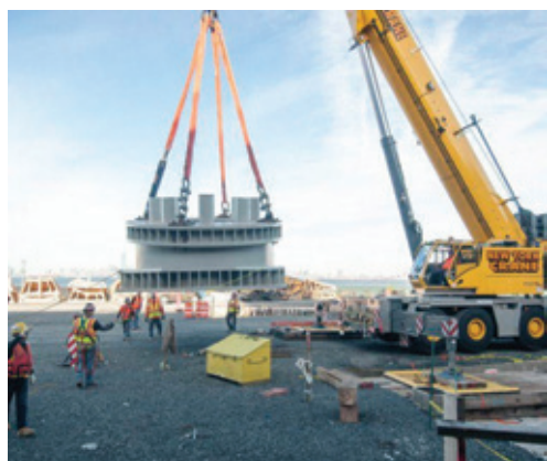
Four steel pedestals, weighing 96 tons each, were lifted into position using a Grove GMK6400.
