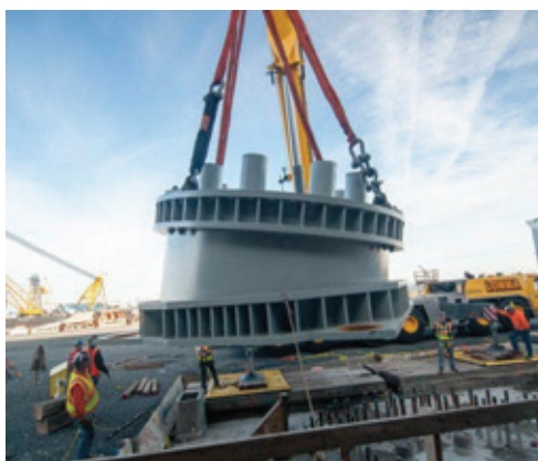
Four steel pedestals, weighing 96 tons each, were lifted into position using a Grove GMK6400.
