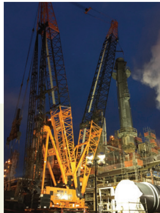
Ness Campbell lifts a 100,000 pound heater stack removal utilizing a Manitowoc 2250 in Max-er configuration and rigging that incorporated an in-house designed halo bar.
