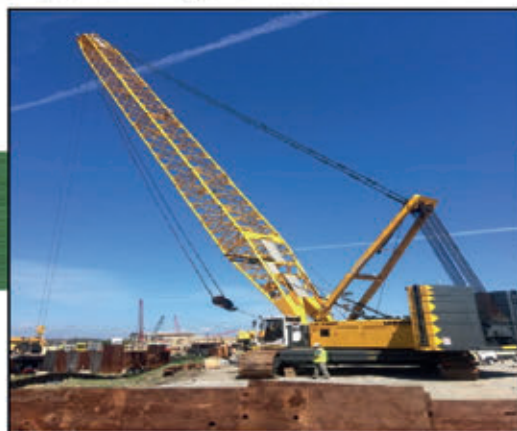
'08 Liebherr LR1300 203' boom, 8' rooster sheave, Liebherr CALL
