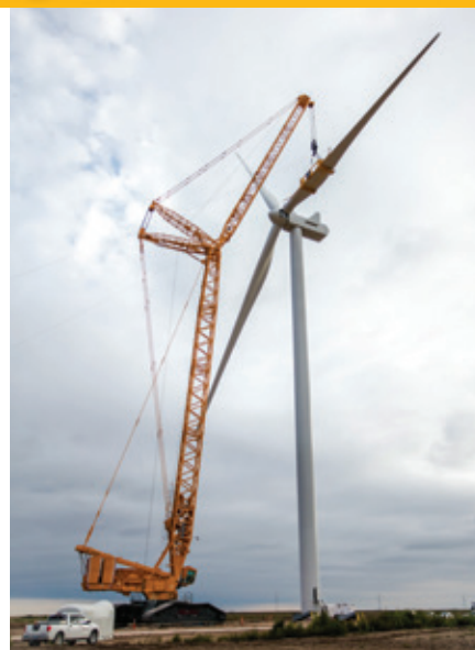
Buckner Companies' LR 11350 completes the erection of a wind tower in Texas.
