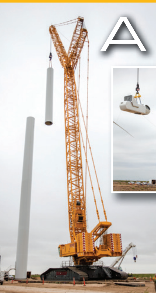
Buckner Companies' LR 11350 completes the erection of a wind tower in Texas.
