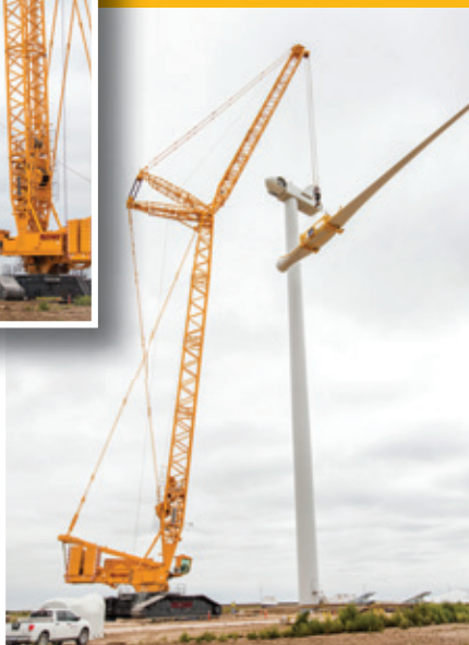
Buckner Companies' LR 11350 completes the erection of a wind tower in Texas.
