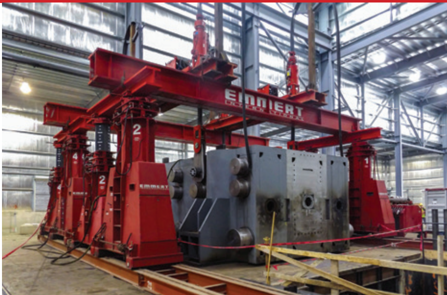
To successfully lift and set the final Krown on the press unit, only six inches of clearance would be available from the top of the strand jack guide to the bottom of the roof structure.
