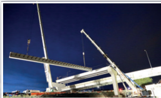
Crane Service Inc. has seven cranes, including six ATs and one crawler, working on the 'Go 10' project in El Paso, TX.
