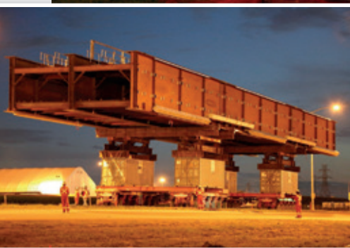
Using Accelerated Bridge Construction, the bridge was set in place before morning traffic.
