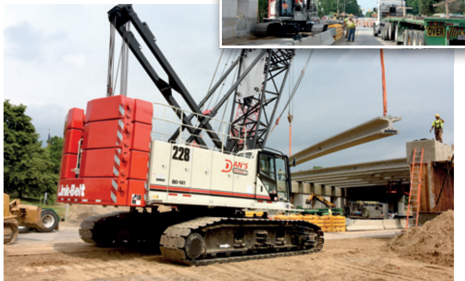
Two Link-Belt cranes, a 248 HSL and a 248 Hylab 5, are placing 144 foot beams for the bridge widening at Square Lake Road.
