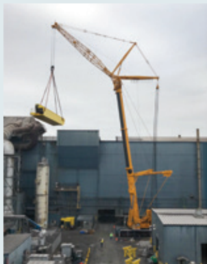
Chellino Crane's Liebherr LTM 1500.8.1 hoists a 130,000-pound overhead crane.
