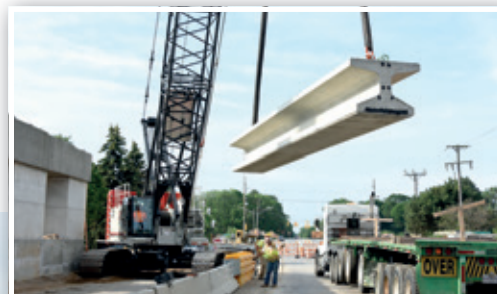
Two Link-Belt cranes, a 248 HSL and a 248 Hylab 5, are placing 144 foot beams for the bridge widening at Square Lake Road.
