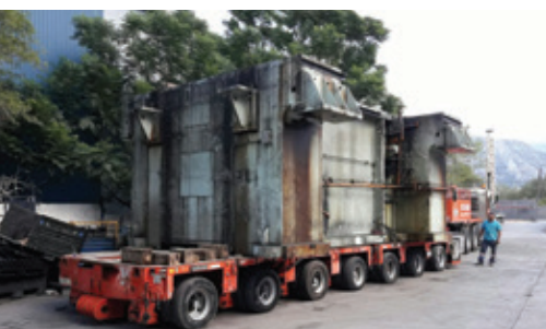
A Tradelossa team rigs in place steam equipment at a Sonora power plant.
