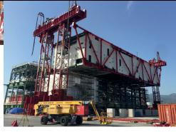
In Phase Three, the module was lowered to 500 millimeters from the top of the foundation. At each stroke, load tolerances were checked by computer, and Fagioli operators proceeded with the lowering operation until the module was at the designed elevation. Thus, the module was ready for the second
