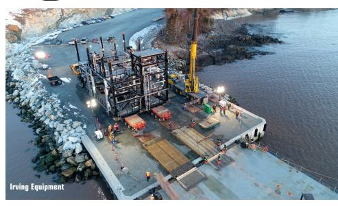
TURNER INDUSTRIES used a unique hookstyle cantilever beam to retrieve a velocity recovery ring from atop a flare structure 208 feet in the air – while the hydrogen flare was still in operation. In only four days, one-of-a-kind rigging hardware was designed and fabricated, and a crane with over 250 feet of luffing jib was built.
