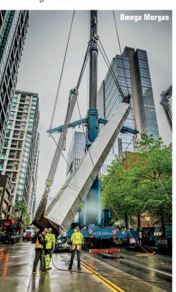
**EMMERT INTERNATIONAL** engineered a custom tower arrangement to lift and set six components - which were lifted 40 feet and traveled 35 feet to foundation pads through a congested work area. Rough set and alignment of each component had to be performed while not interfering with existing building structure. No other work could be obstructed for installation.
