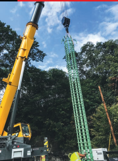
The 100-ton capacity Grove GRT8100 features a 39.2 to 154.3 five-section full power boom.
