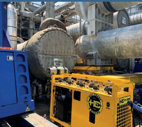
Both heat exchangers weighed in excess of 250,000 pounds. They were loaded onto the HT500 system and engineered support stands.
