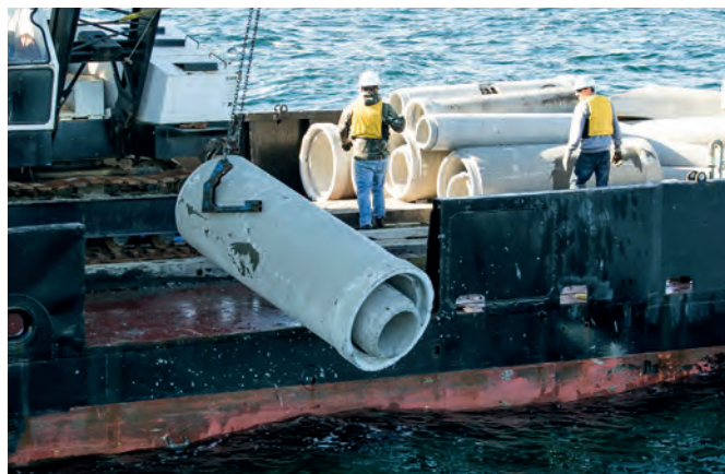
Fassi cranes will be used in the construction of artificial reefs.
