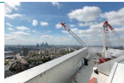
ALE's Lightweight Service Crane lifts a BMU in London.
