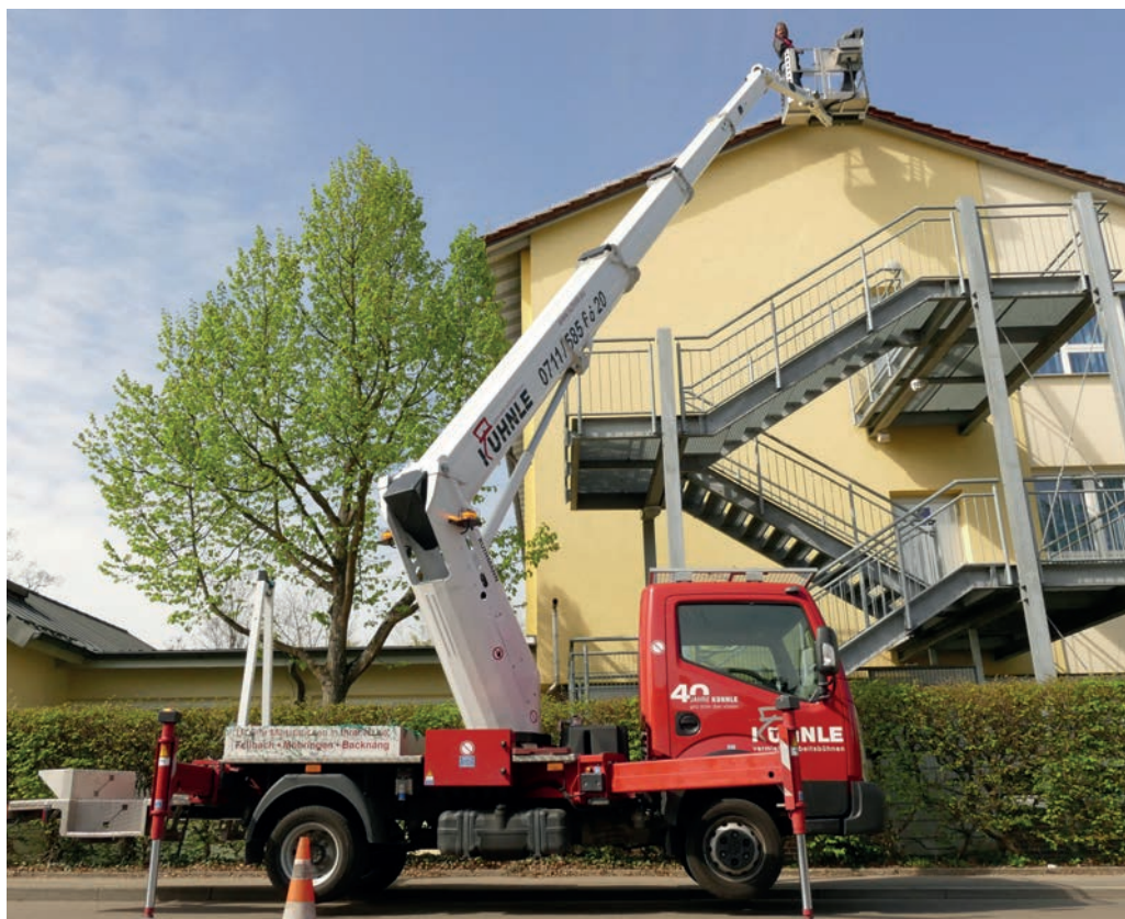
A facility management company in Germany has rented platforms from truck mount specialist Kuhnle, based in Fellbach near Stuttgart, to protect a 15-store DIY chain from damage caused by pigeons. The deal was organised through PartnerLift, the national cooperation of more than 100 rental companies.
