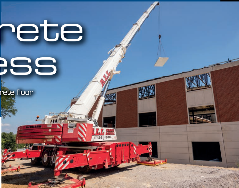
ALL's 265-ton capacity Liebherr LTM 1220-5.2 was rigged with a 197-foot boom and the Liebherr VarioBase system.
