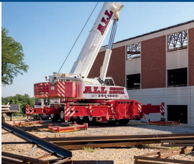
Because the exterior walls had already been set, the crane had to be positioned outside the building, and the operator was unable to see where he would be setting the floor pieces.
