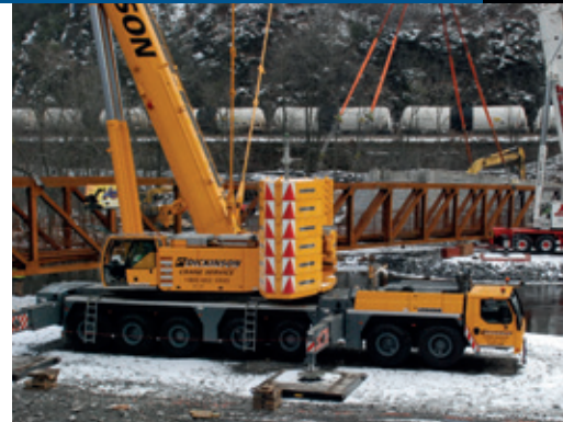
The Liebherr 1400's chassis elevating feature allowed it to maneuver past several rock outcroppings.
