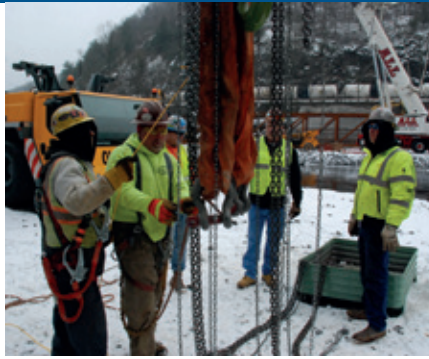
Rigging the bridge sections was complicated. It took several hours to balance the loads and set the chain-hoists to their proper heights until the bridge mating could start.
